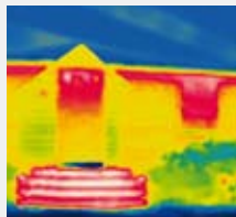
Building: Heat Loss
